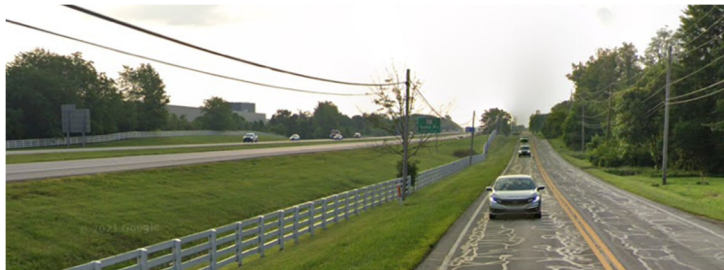
Image of Old S.R. 161 (E. Dublin-Granville Road) with adjacent 4-lane limited access expansion – new S.R. 161.
