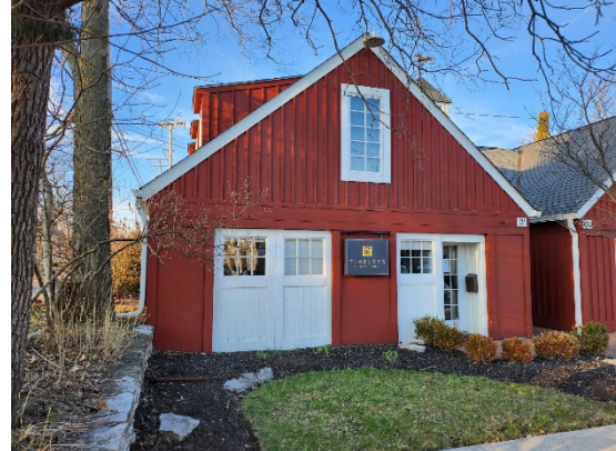
Commercial Retail Building Dublin Ohio
