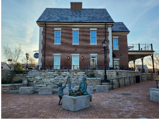
Commercial Restaurant Building Dublin Ohio
